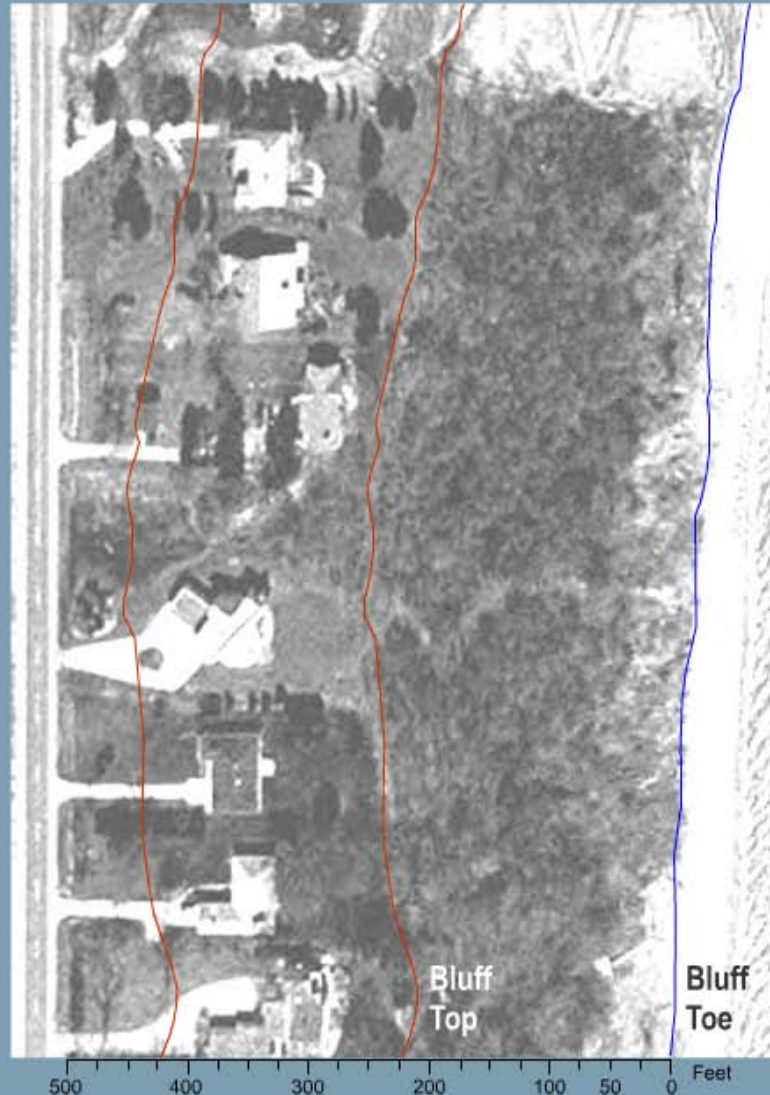
The bluff material for the area in the image above consists generally of glacial till (cohesive soils) and averages about 113-ft high (greater than 30-m). The current slope in this area measures 24-degrees.
