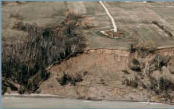
High (>100 ft), complex bluff that failed in the early 1990s by a large deep-seated slump north of Milwaukee, Wisconsin, on the western shore of Lake Michigan.
